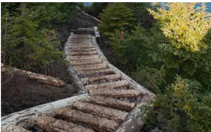
Stairs built out of timber and filled with granular (Newfoundlander)
