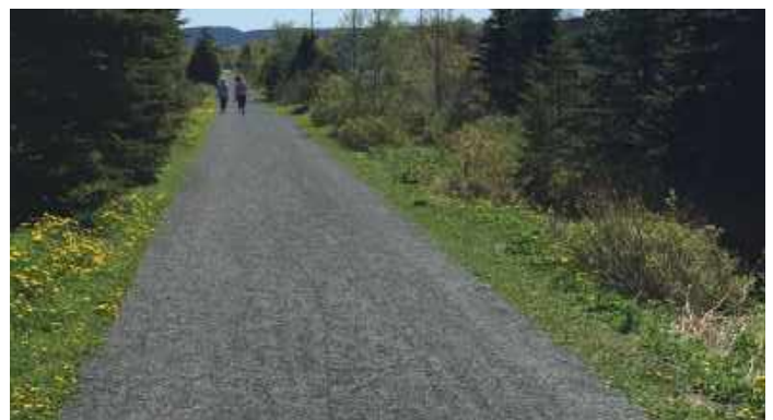
Level, well-graded granular trails can meet accessibility guidelines, trails do not necessarily have to be paved (City of Mount Pearl)
