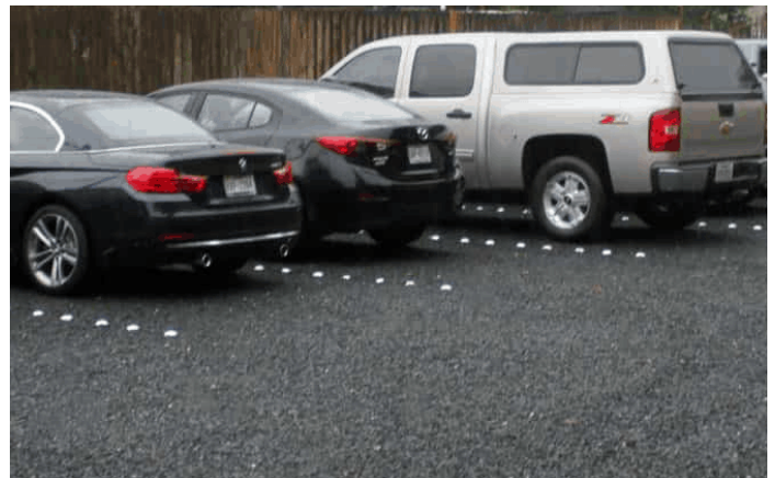
Pavers set in granular to delineate parking spaces (Truegrid Pavers)
