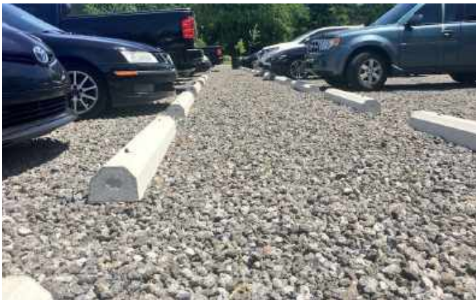
Precast concrete curbs used to delineate parking spaces in a granular parking area (Pinterest)
